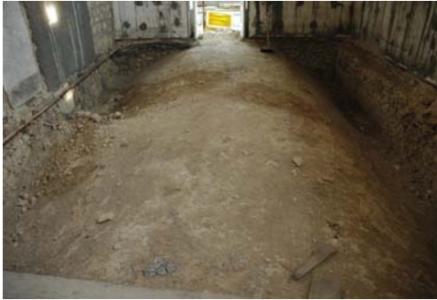
Figure 5. Some vaults details.
