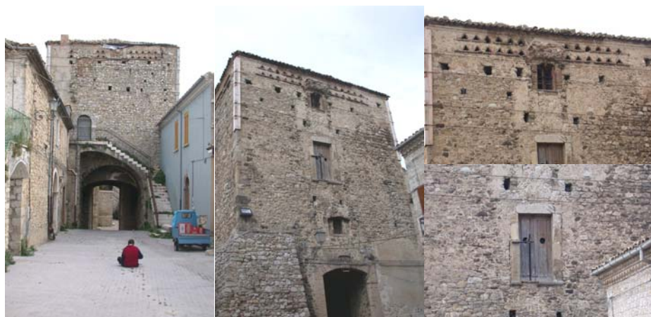
Figure 4. The old Castle Tower.
