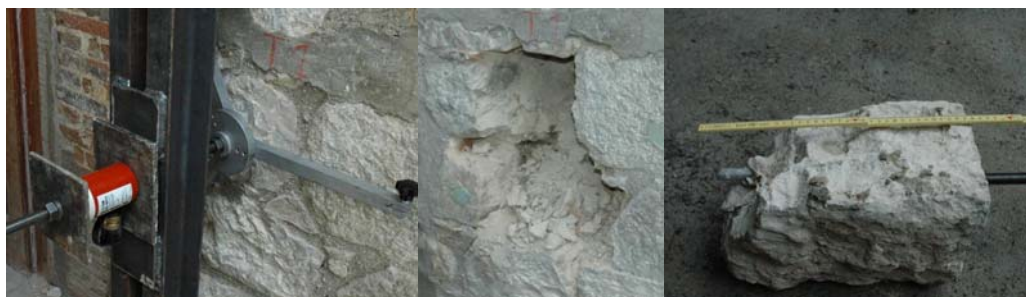
Figure 9. Shear pull out tests.
